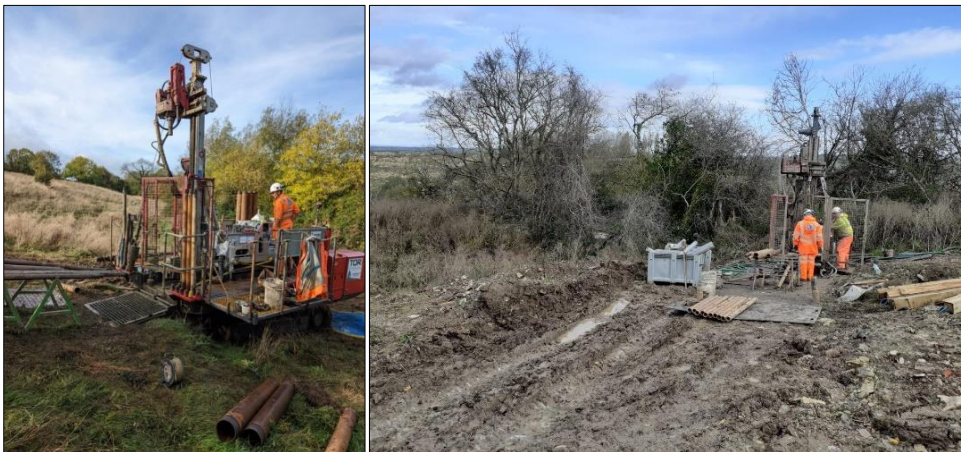
A detailed ground investigation with boreholes was undertaken to help design the remedial measures
