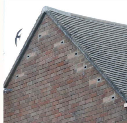
'Universal bricks' integrated within the building's fabric
